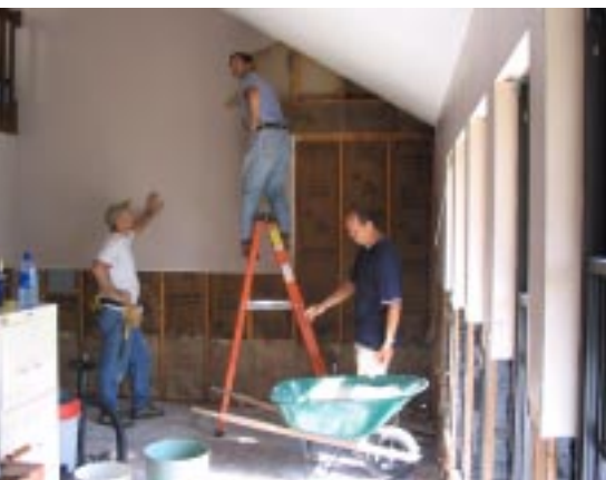
We Care chaplains assist We Care Associate Jim Britnell with hanging sheetrock in his family's living room after their home suffered extensive water damage from Ivan
